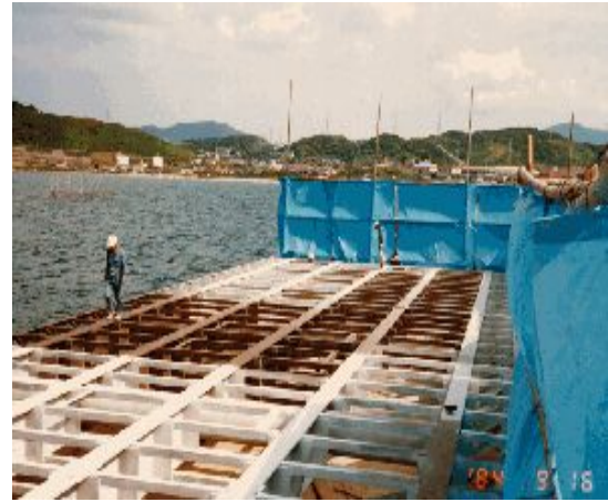
図一５ 栈橋床版設置用桁
